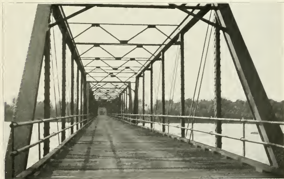
NEW STEEL WAGON BRIDGE, MONROE
